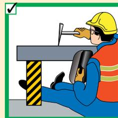
◀ As with jacks, never place any part of your body under the load. Load must be on cribbing before venturing under.
