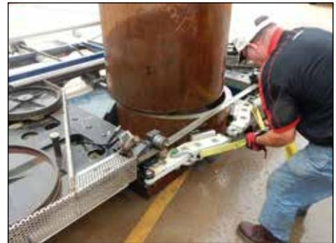
▲ Pipe cutting with BS portable band saw.
