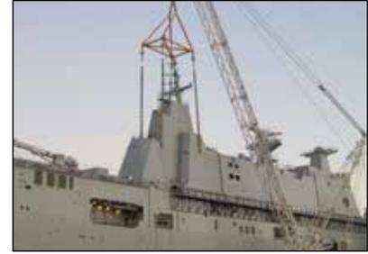
Synchronous hoisting and load positioning
