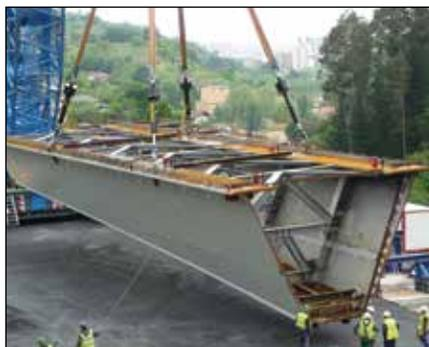
▼ Rigging engineers used the SyncHoist system to precisely monitor and adjust each lifting point independently, or together in a synchronized manner to position the 1140 ton nuclear plant module.
