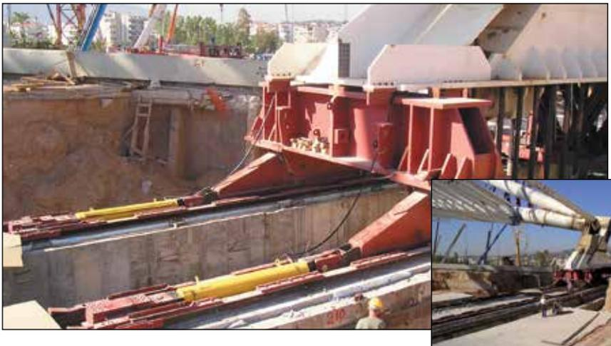
▼ RR-cylinders provide power and precision in a special hydraulic press.
