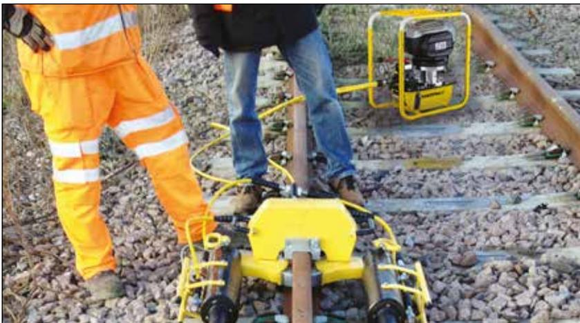
◀ Special Enerpac ZC3-Series pump used for rail stressing applications.
