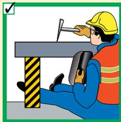
◀ Never place any part of your body under the load. Ensure the load is on a solid support before venturing under.
