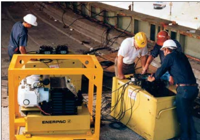
◀ With similar specifications, a gasoline-powered EGM8000 Series is shown here performing a synchronized lift.
