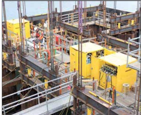
▲ *Custom hydraulic pump for a bridge deck launching system.*
