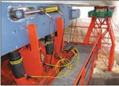
◀ Custom cylinders used for incremental bridge launching systems.
