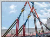
Custom SyncHoist cylinders for placement of stadium roof trusses.
