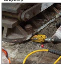
Maximum system pressure must be limited to half the rated pressure (5000 psi)
